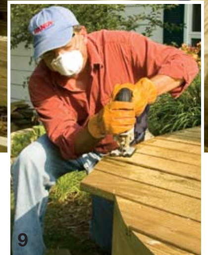
Trim the deck boards with a jigsaw to follow the face of the plywood fascia.
