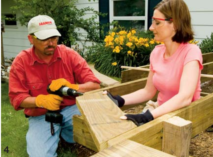
Fasten scrap lengths of 2x8 material between the joists to serve as headers.
