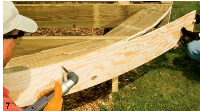
Use a jigsaw to cut the header sections along the curve (left) and cut away any sections of beam that protrude past the joists. Soak the plywood for about an hour to increase its flexibility; then slowly form it around the curve (above).
