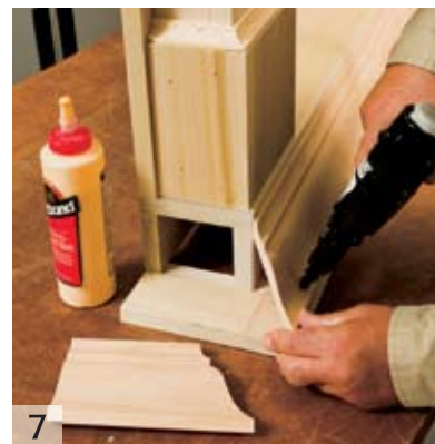
Attach the crown molding to the mantel with glue and 1-1/4-in. brad nails.
