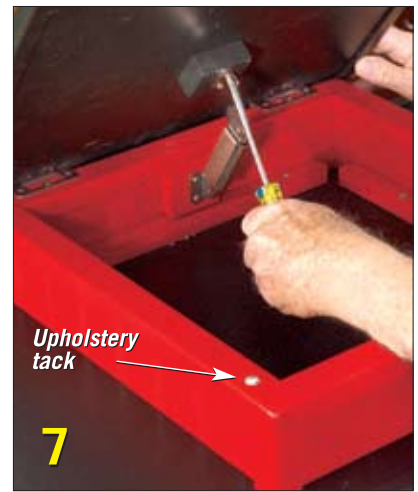
Install the spring-loaded lid supports (see SOURCES ONLINE). These supports provide resistance when you open and close the lid. Various spring strengths are available to accommodate different lid weights.
