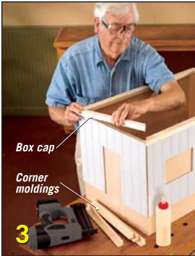
Attach the box caps and corner moldings. Miter the box caps to fit around the top edges of the main and small boxes. Attach the box caps and corner moldings with glue and 1-1/4-in. brad nails.
